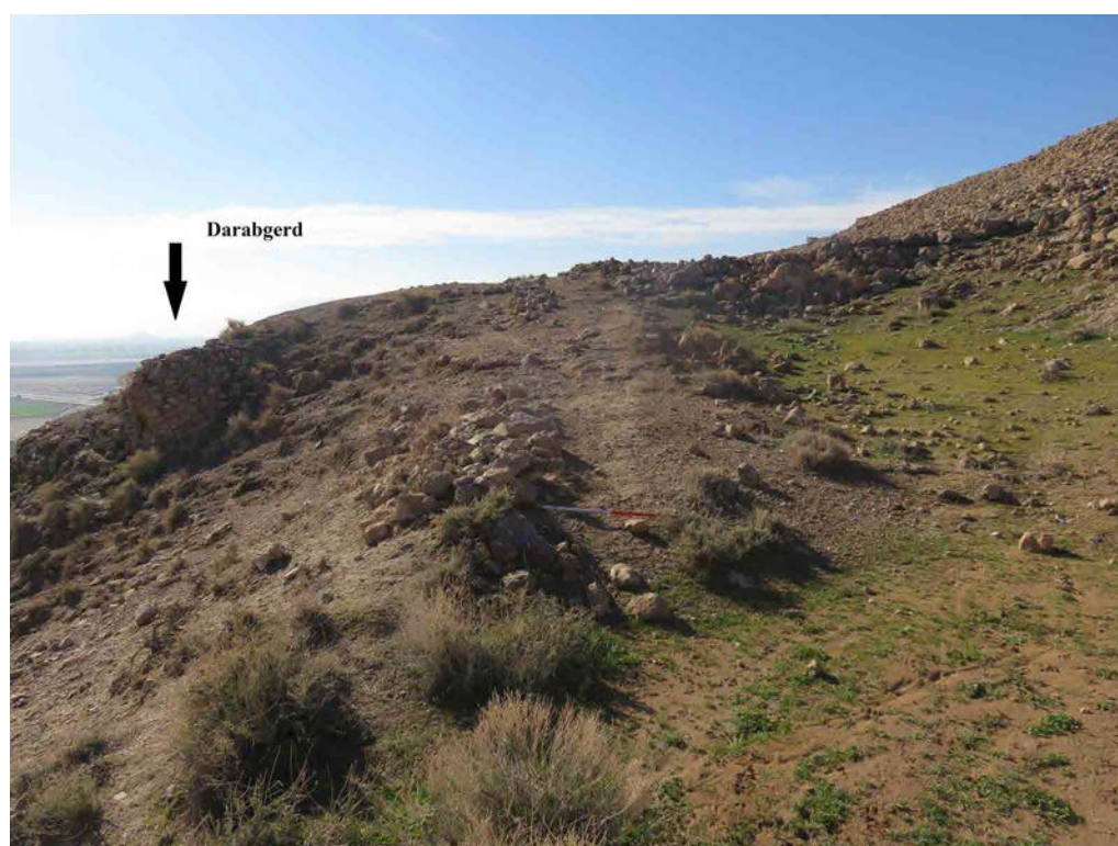
Fig. 11: Remains of the wall and tower of Shahneshin-e Korsia Fortress, and the view of the city of Darabgerd from atop this fortress (Authors, 2024).
