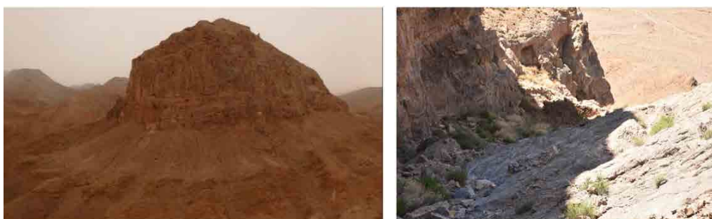
Fig. 3: Gerdkūh: Left- View of Gerdkūh from the southwest (Saber, 2023: 50); Right- Dam on the northern slope (Authors, 2024).
