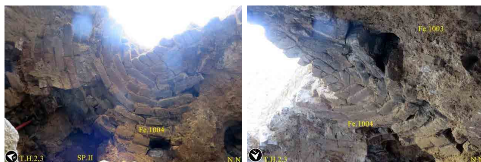
Fig. 15: Part of the brick dome or vault of the tomb and the vaulting technique in the Naqqārechi tomb (Janjan, 2022).
