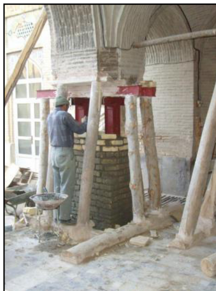
Reconstruction of Pillar
