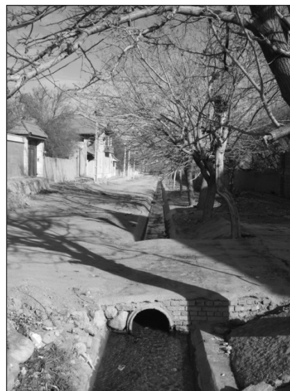
Main Runnel of Taft Qanat in Yazd
